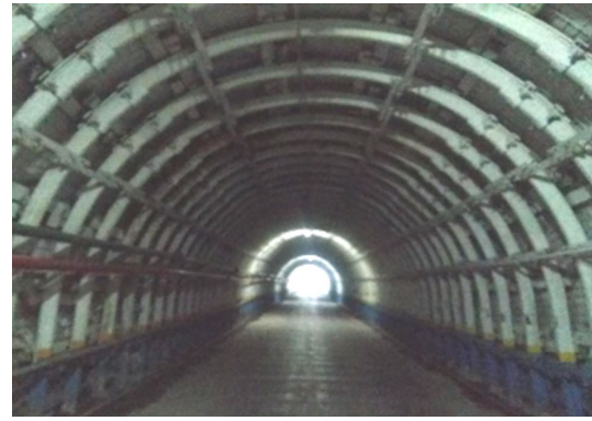
Fig. 10 Site image of the U-shaped steel supports after construction
