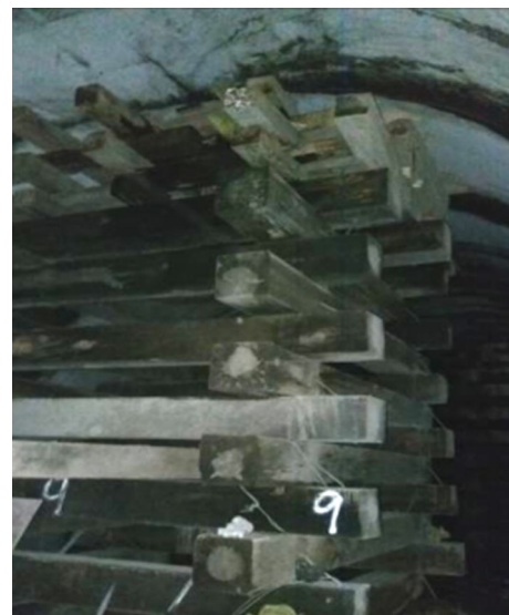
Fig. 5 Image of the crib construction field
